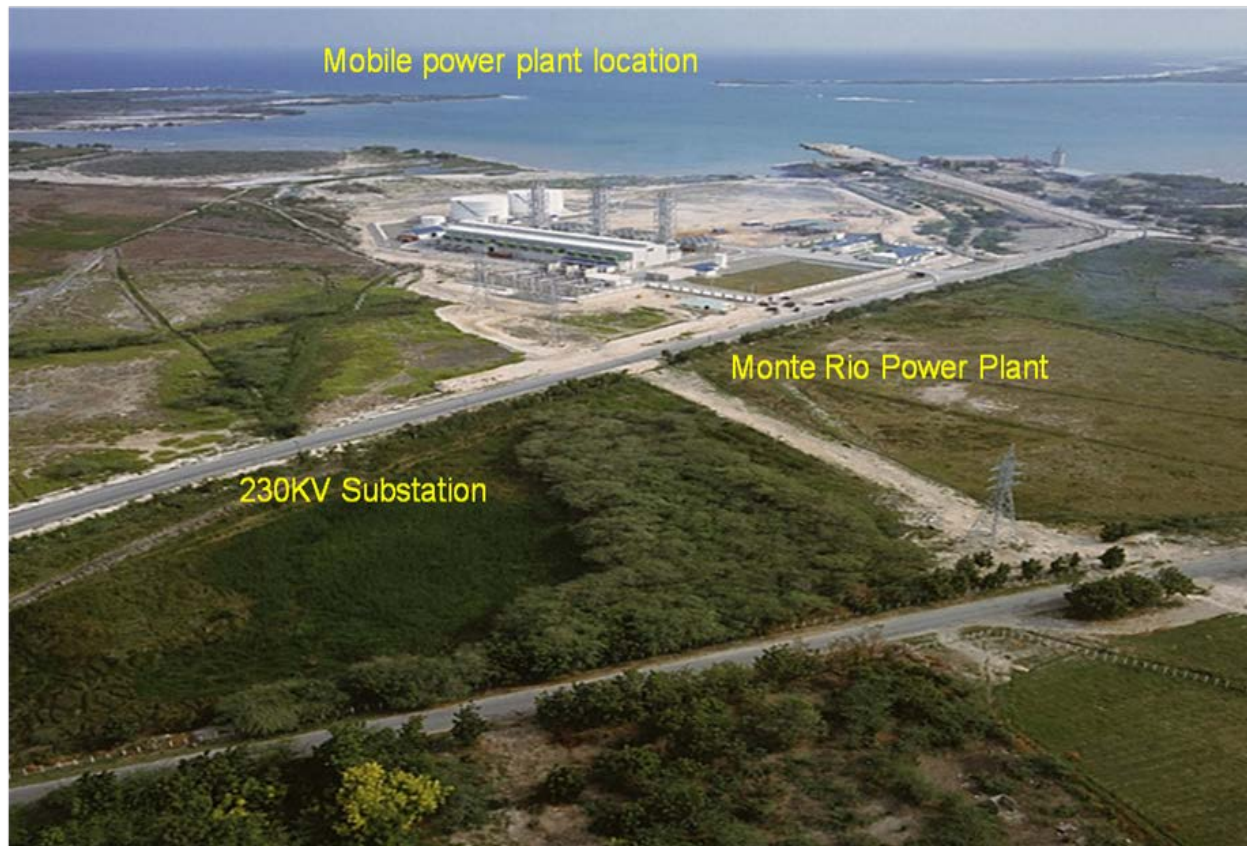
Figura N° 5.33.- Monte Rio Power Plant (100 MW)
