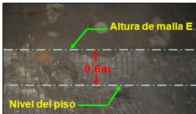
FIGURA 5.23: ALTURA DE LAS MALLAS SOBRE LAS CAJAS
