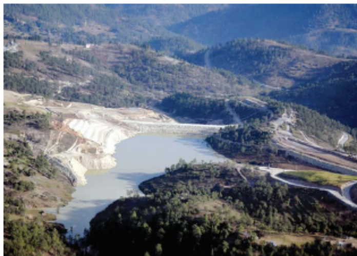
An aerial view of Marlin mine's tailings impoundment. With the safety and well being of the land, waters, and population in mind, Marlin mine is highly committed to operating an ultra-safe and environmentally sound mining operation. The new multi-phase cyanide and metals removal plant will help ensure that it continues to do so.
