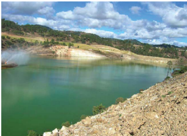
The tailings water generated from the milling operation is treated with an air cyanide removal technology prior to discharge to the mine's tailings impoundment. The impoundment currently has a capacity of 4 million m 3 and is expected to expand to nearly 20 million m 3 by the end of the mine's life.
