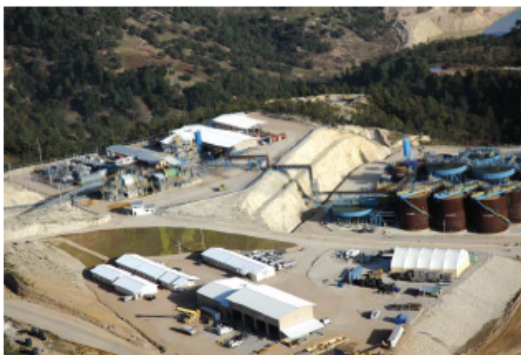
The Marlin gold mine, located in the western highlands of Guatemala, is a combination of open-pit and underground mining with a conventional milling operation that began commercial production in the fourth quarter of 2005. The mine is owned by Montana Exploradora de Guatemala, S.A., a wholly-owned subsidiary of Goldcorp Inc. The mill is designed to treat a minimal 1.82 million metric tons of ore per year.
