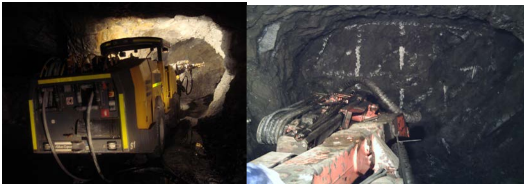
FIGURA 19: PERFORACION DE AVANCE (Izq: Rocket boomer S1, Der: Monomatic)
