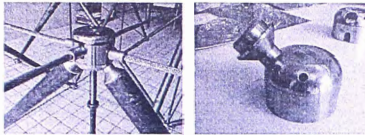
Fig. 2.26 Tomado de: René Motro, Libro: Tensegrity Structural Systems for the Future, Assembly at node
