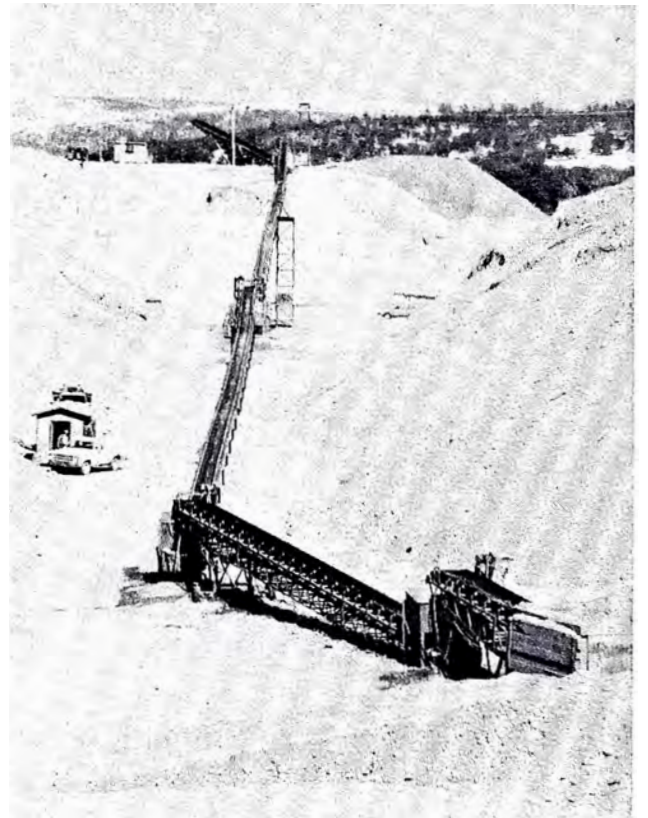
$7 million was spent to reconstruct the Yuba No. 21 dredge. It now excavates alluvials down to 140 ft below pond level.
