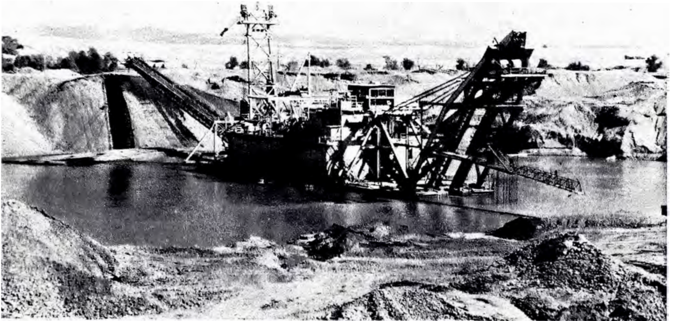
$7 million was spent to reconstruct the Yuba No. 21 dredge. It now excavates alluvials down to 140 ft below pond level.
