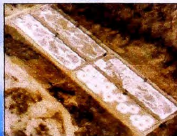
AEROBIC BASINS AND DIGESTERS
