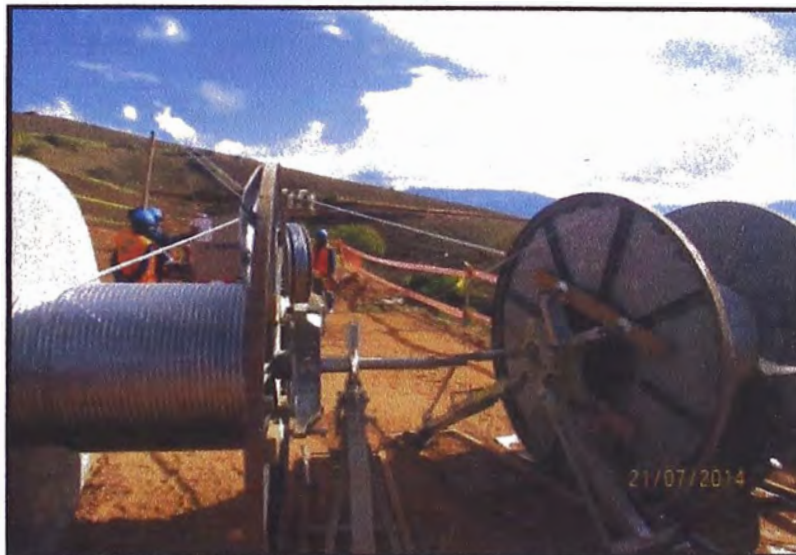
Figura 3.23: Tendido de conductor
