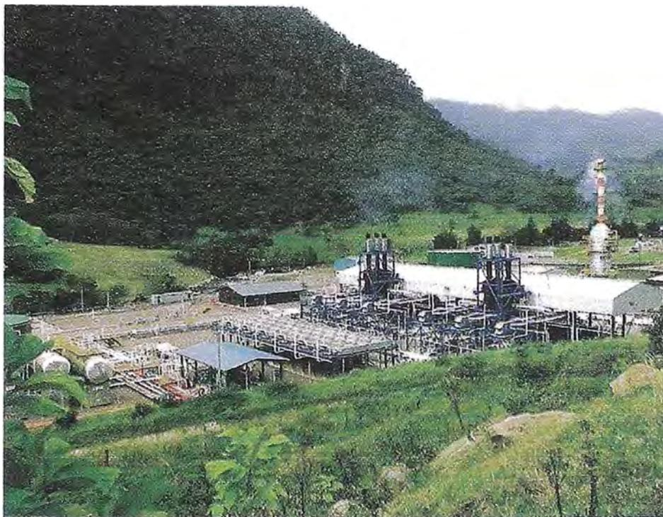
The Paramo Pump Station for Oleoducto de Crudos Pesados, Ecuador, is equipped with six Wärtsilä 12V32LN pump sets.
