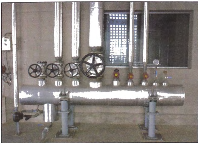
Figura 3.35 Manifold Principal
