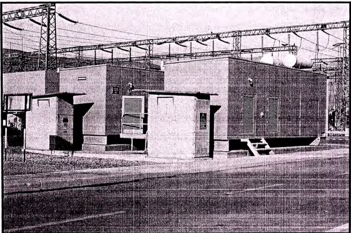
Figura. 2.25. Generadores Diesel (Black Start)
