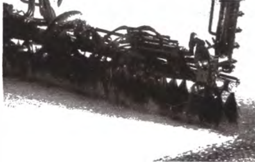
◀ Spraying asphalt
