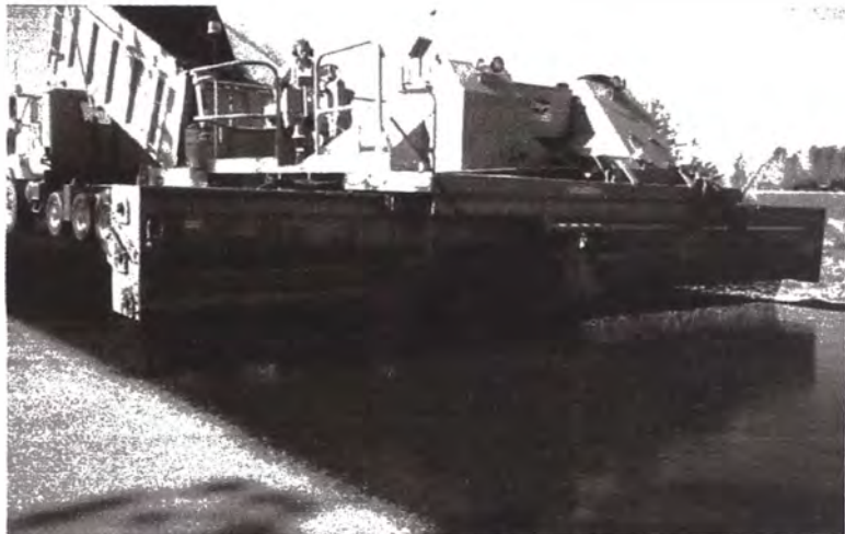
▲ Spreading cover aggregate
