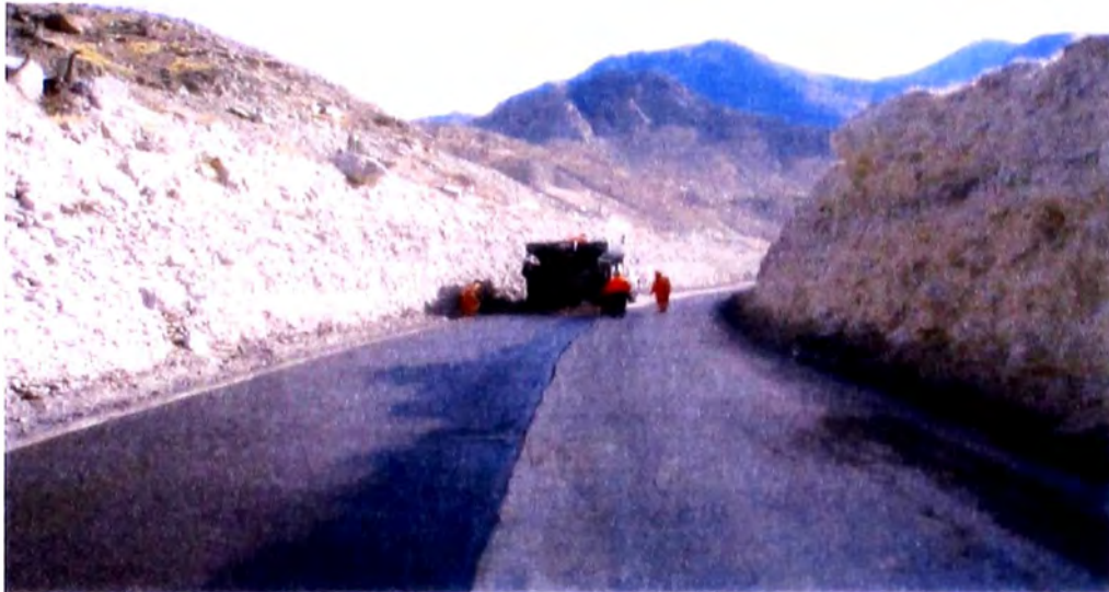
FIGURA N°2.8 TRATAMIENTO SUPERFICIAL SLURRY SEAL.
