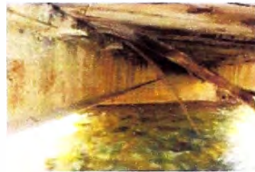
Viga Interior (VM-01)
