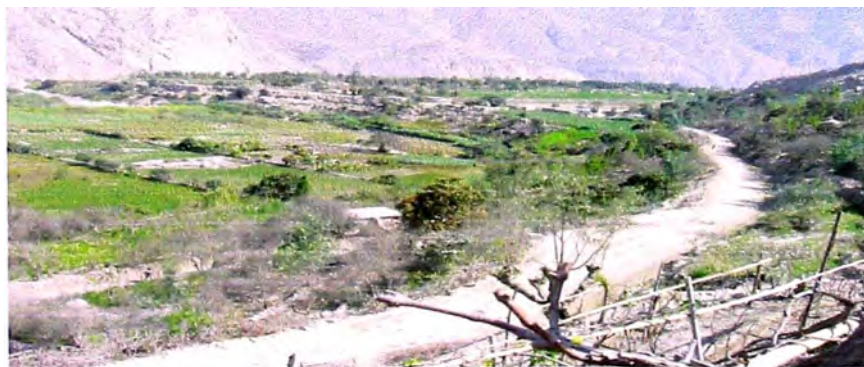
Carretera Cañete – Yauyos (tramo 58+800-59+100)
