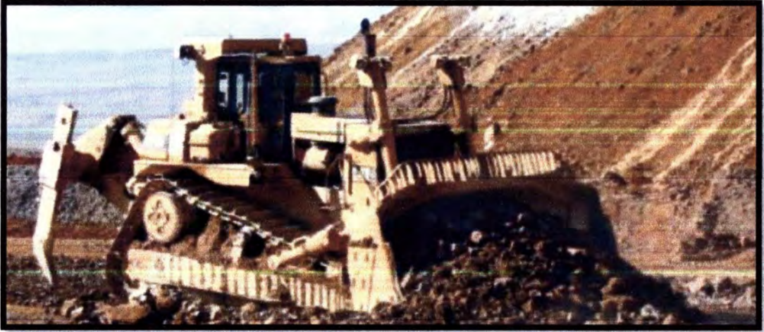
FIGURA 9: TRACTOR ORUGA REMOVIENDO MATERIAL
