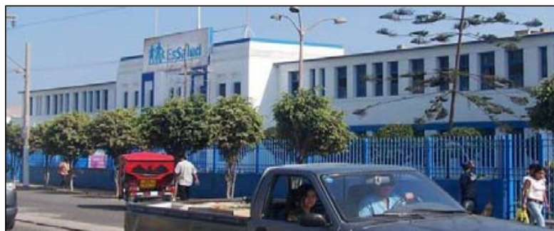
Figura N°6.18 Hospital II, ESSALUD, San Vicente de Cañete
