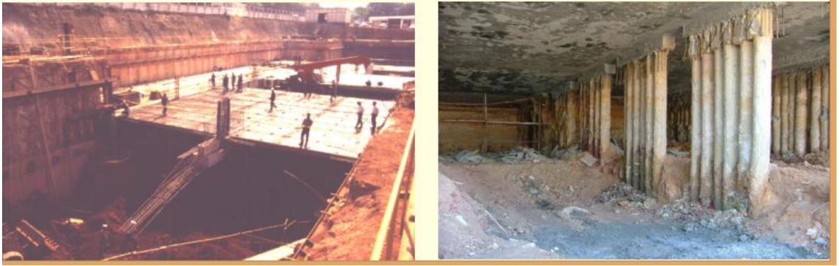
Figura N°2.38 Cut and Cover, Excavación Inversa – ITA
