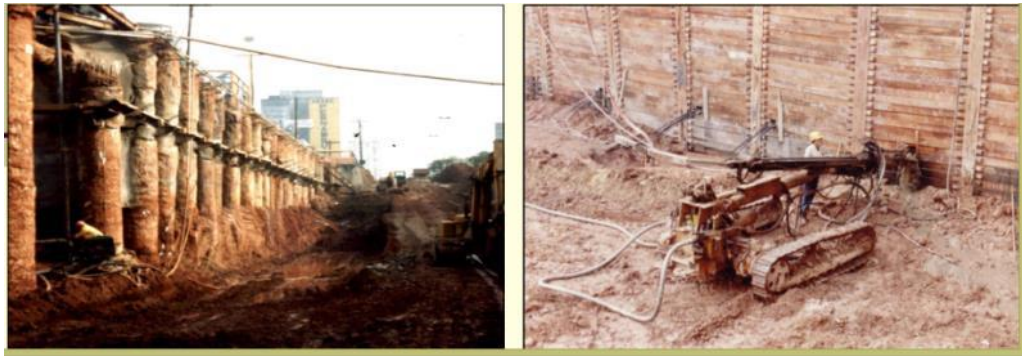
Figura N°2.49 Sostenimiento Amarrado (Tie-Backs) – ITA
