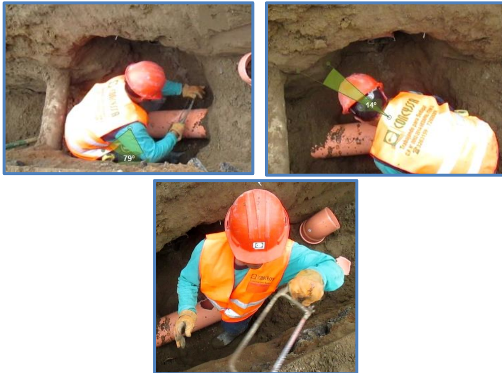
Figura N°26: Corte circular de colector
