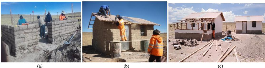
Fig. 2: Views of part of the construction process of the experimental modules, (a) adobe walls, (b) fiber cement roofs, and (c) wooden structure of the attached greenhouse (at ME2).
