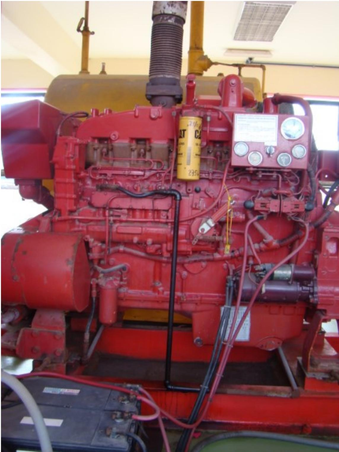
**Figura 51***Bomba contra incendio P-202*
