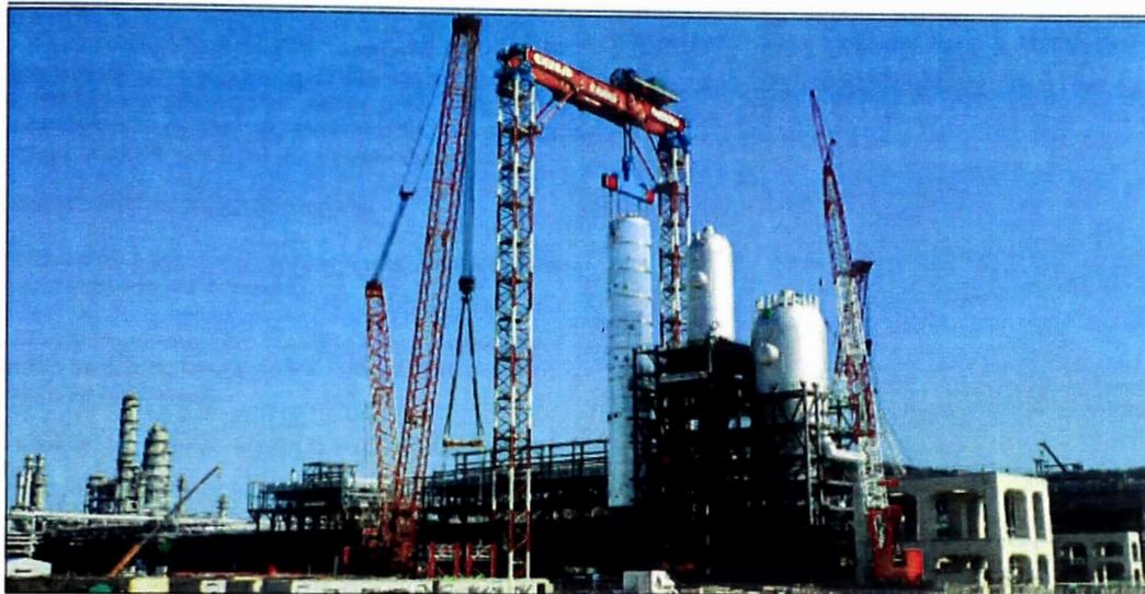
Chunjo- Fagioli , a Korean joint venture between Chunjo corporation and Fagioli, performed really innovative heavy lifting operations at the petrochemical plant in Yeosu, South Korea: No.4 Vessels up to 870 ton were lifted, skidded and installed inside their plinths by means of a new concept "traveling mega gantry system" 94.4m high and 40m span.
