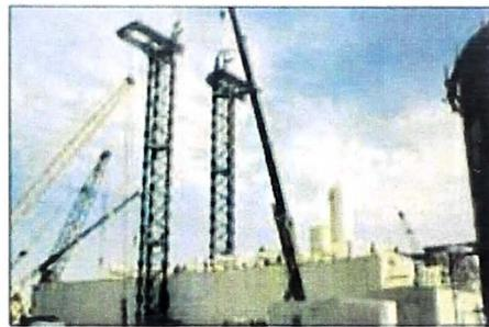
The lift arrangement comprised of a pair of 36 metre high triangular format Towerlift supports. An L300 jack was mounted on a cantilever beam at the top of each tower, with the tie-back forces provided by an L50 jack for each beam. The L300 jack cables were then attached to the lifting trunnions by the use of fabricated link plates.
