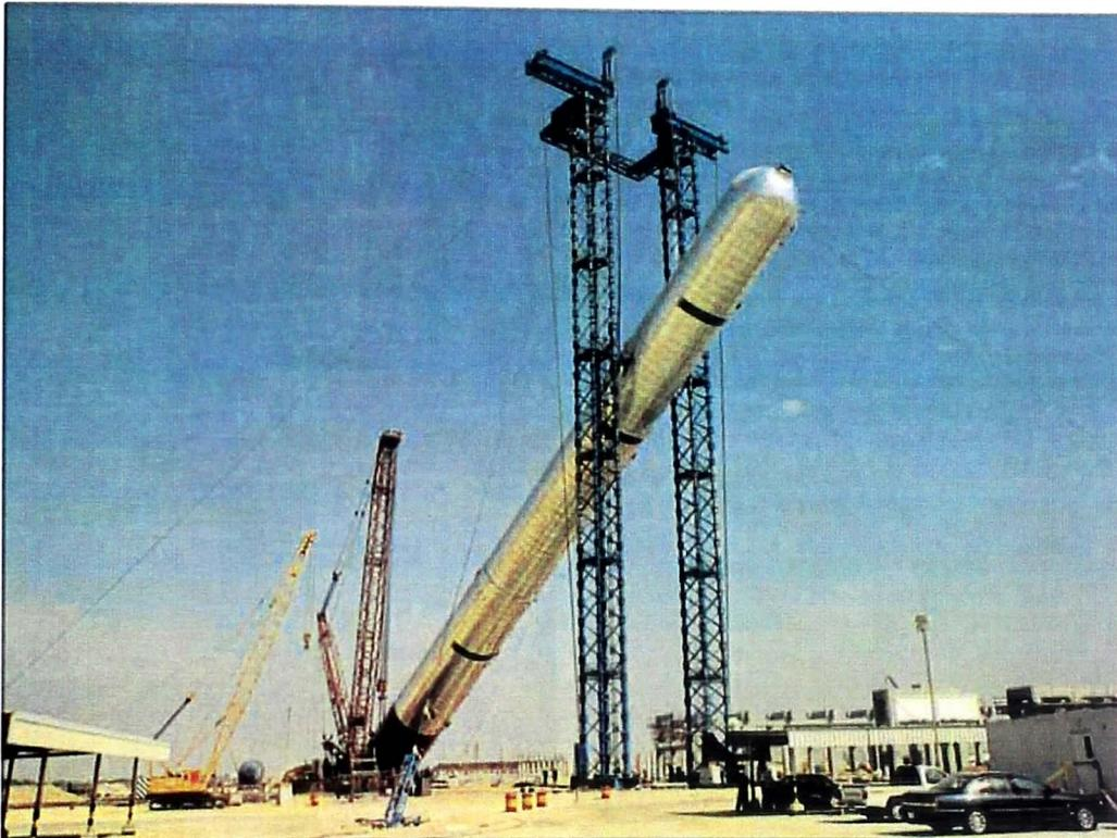
The erection of a 104 metre tall Splitter vessel was carried out by Fagioli PSC at a new Polypropylene facility being constructed for the Saudi Polyfins Company.
