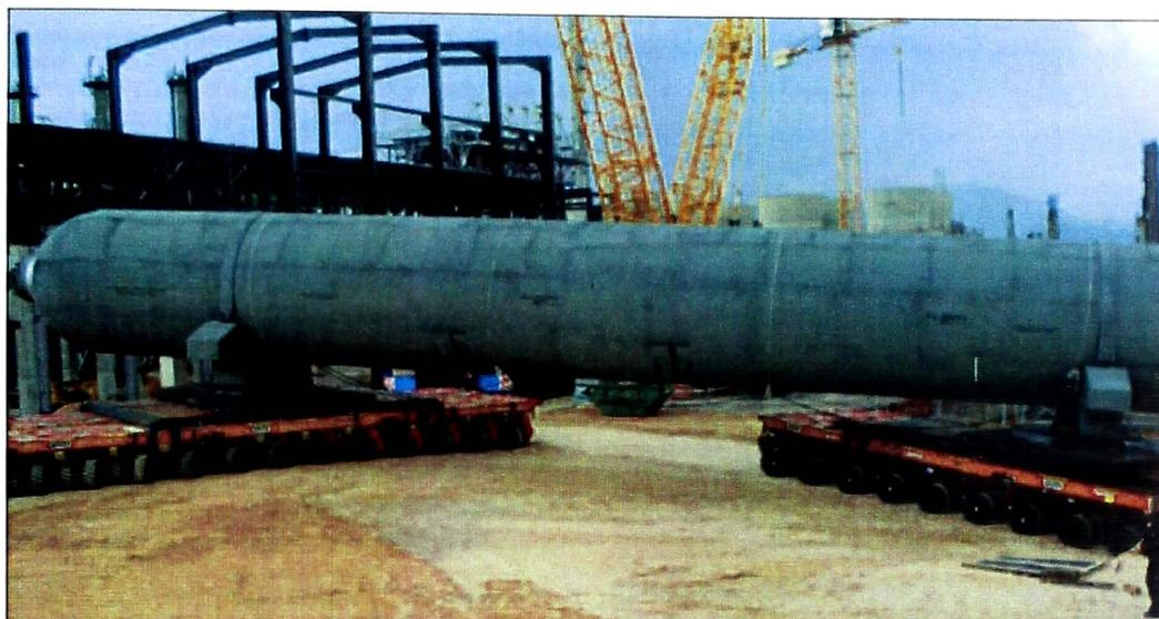
Above: Transport of the heaviest vessel by means of 2x12 and 2x 14 SPMTs axle lines
