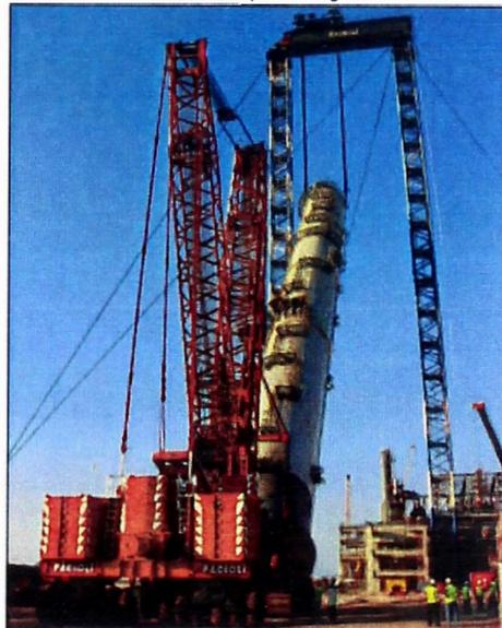
In July 2009 the deethanizer (7 m in width and 600 t in weight) was lifted using our tower lift and strand jacking system. Talling was carried out using a tailing frame connected to the vessel and attached to Fagioli No.2 x 12 SPMTs axle lines.
