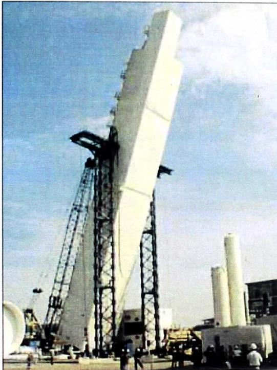
Fagioli PSC were awarded the contract to lift a 65 metre long Cold Box weighing 450 tonnes, and a 25 meter long Heat Exchanger Box weighing 180 tonnes, during the construction of an Air Separation Unit to supply oxygen to the Copper Smelting Plant being built at Gresik, near Surabaya. The first stage of the contract was to lift this 450 tonne Cold Box.
