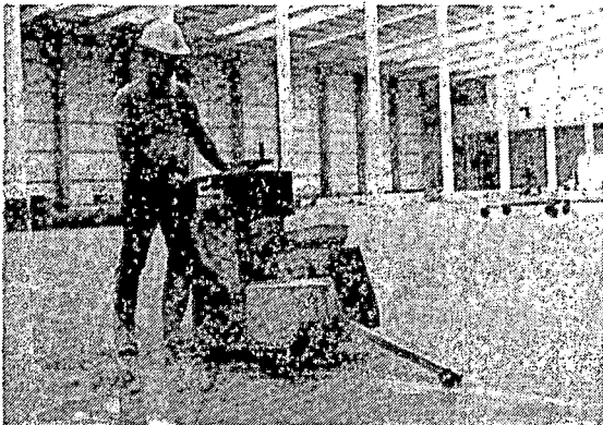
Fig. 6 Wet cut saw induced joints are far less prone to breakdown than pre-formed construction joints.
