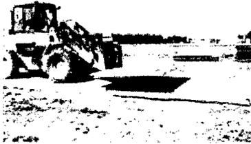
while the loader rests on the previously placed mats. In this case, the installer must stand in front of the loader on a previously laid mat and thread the positioning bar through the mats to align them. The installer must remain in view of the equipment operator at all times, particularly during this type of installation. Observe strict safety standards when performing this procedure.
