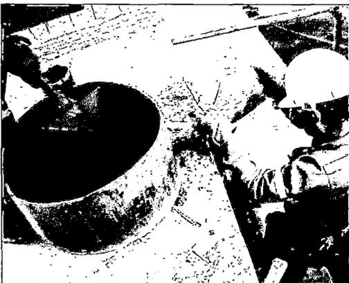
A black and white photograph showing a person pouring grout from a bucket into a formwork box. The grout is being poured from a height, and the person is wearing a hard hat.                              |
