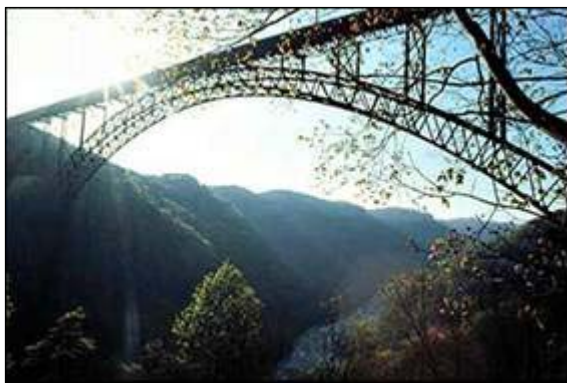
(c) Puente New River Gorge.
