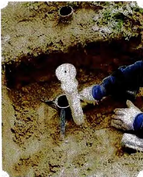
**Photo 5. Placing ring extension on top of ring**
