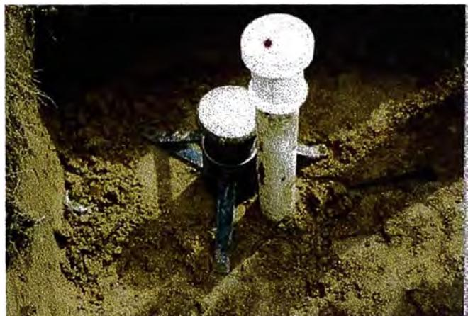
**Photo 6. Placing top on ring extension ready to hit with mallet**
