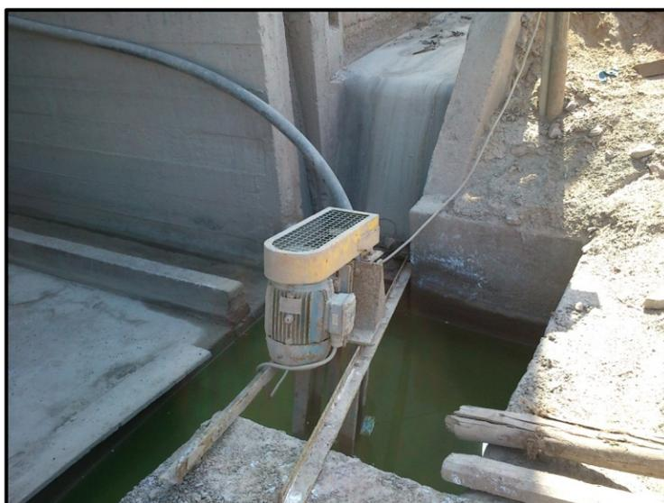
**Figura 4.6:** Bomba vertical de pulpa 2"x2"
