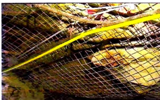
Figura 3.16. Cable Leaky Feeder
