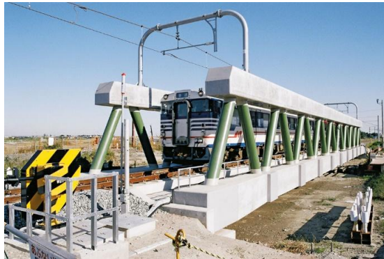
(c) Puente Yamaguragawa
